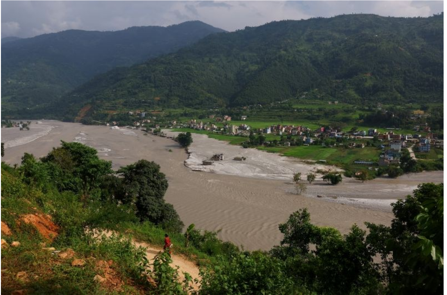
The remains of damaged houses stand on the banks of the Trishuli River, following the deadly flash floods and mudslides, in Nuwakot district, Bagmati province, Nepal, September 8. REUTERS/Anushree Fadnavis
